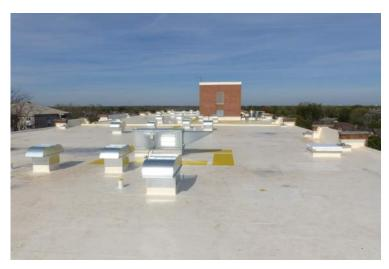
St. Regis Condominiums is a 90-unit residential building located in Lombard, Illinois. The building is a 7-story structure with cast-in-place concrete floor slabs and columns. The main roof of the building and the penthouse roof total approximately 18,000 square feet, and originally consisted of a low-slope built-up system with internal drains.
